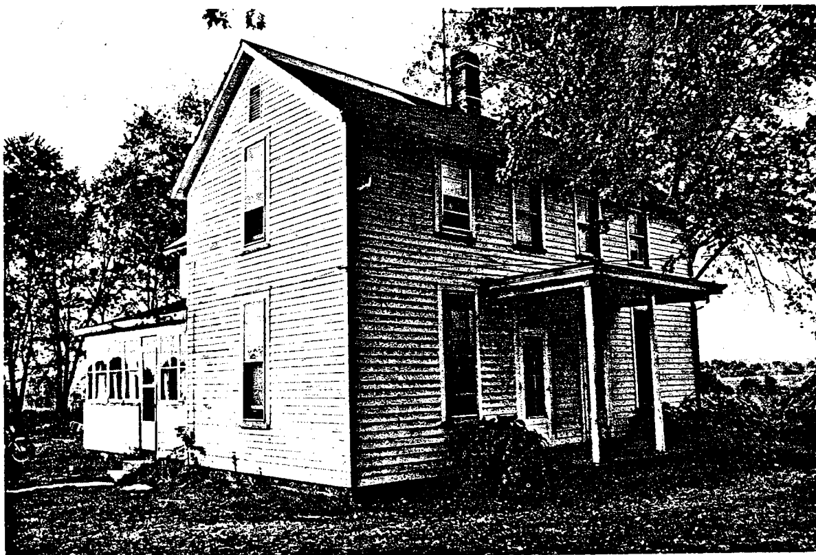
Figure 15.—Test structure 19, near a coal mine.
