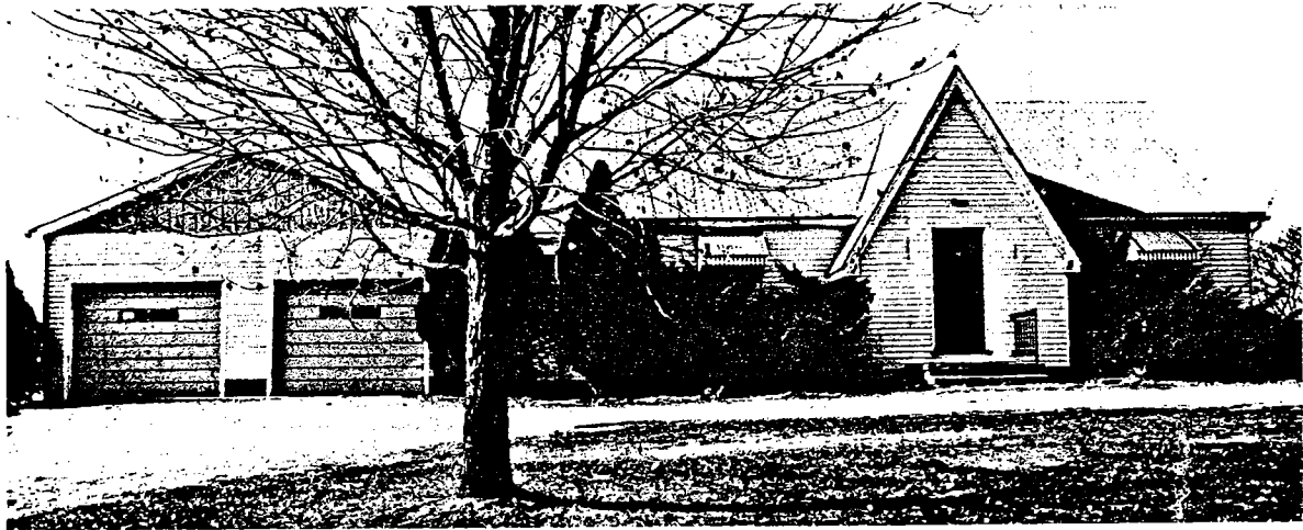
Figure 16.—Test structure 20, near a coal mine.
