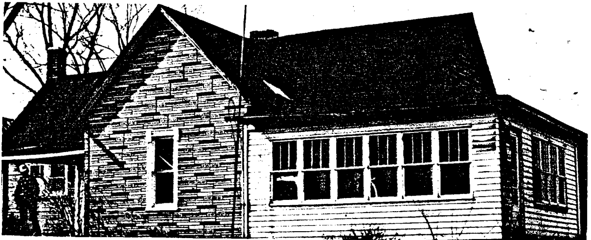
Figure 21.—Test structure 27, near a coal mine.
