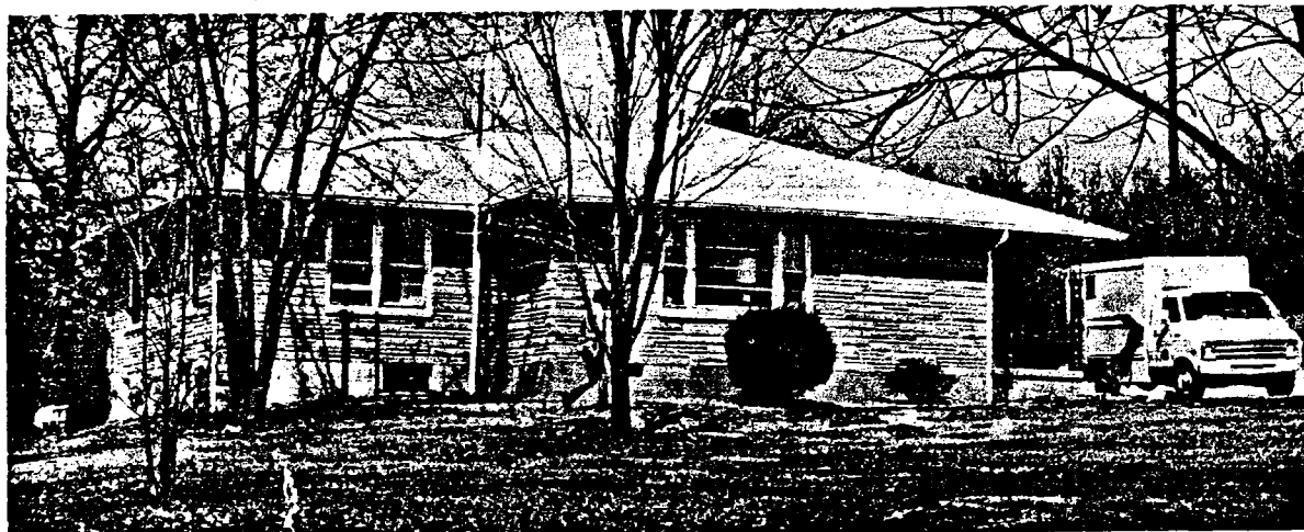
Figure 24.—Test structure 30, near a coal mine.
