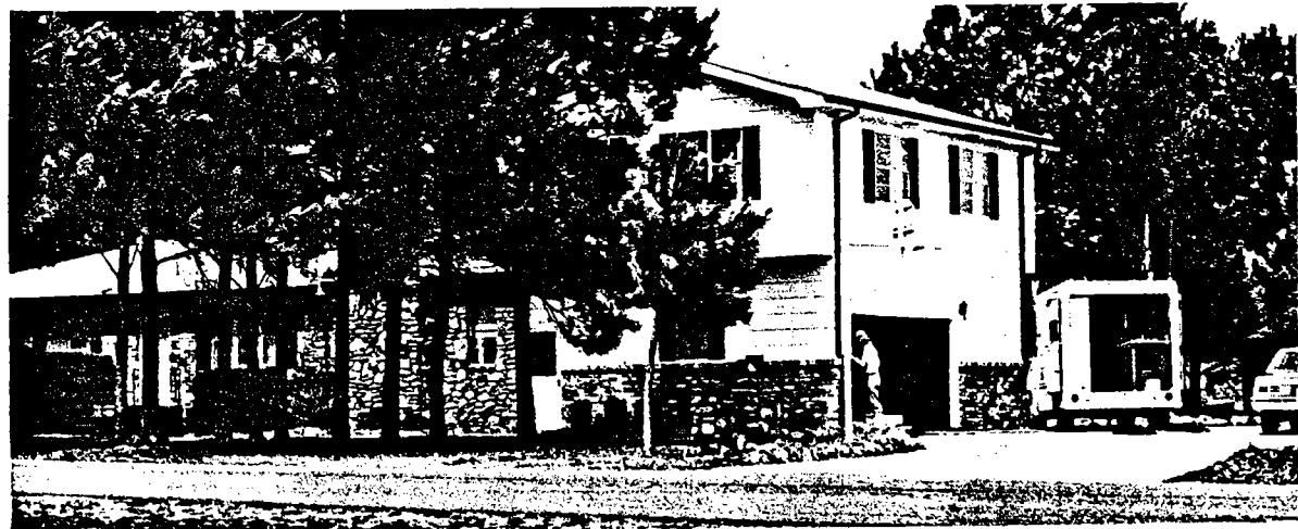
Figure 18.—Test structure 22, near a quarry.
